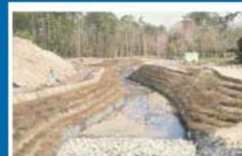
Figure 6. A VRSS structure immediately after construction
